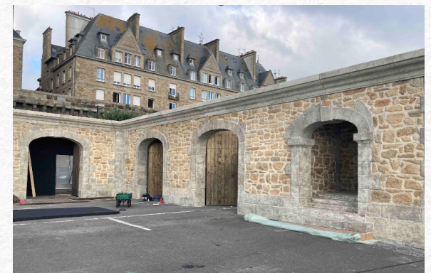
Staff and textured polystyrene facade for the Benjamin Franklin series. Head Production Designer Dan Weil, production : Apple TV, 2024. © Gilles Bontemps
